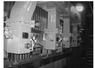
*New side wall OFA was installed on this combination waste wood and oil fired power boiler.*
