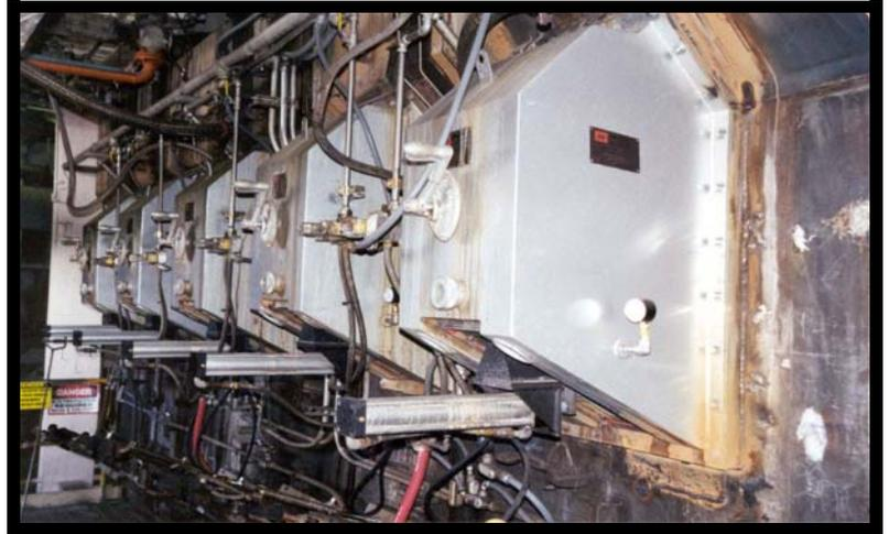
The new secondary air nozzles were placed on the left and right side walls (with five air nozzles on each side) and one nozzle on each the front and rear walls. This arrangement provides for a slight but effective rotational component to the secondary air delivery, which is beneficial in reducing carryover.
