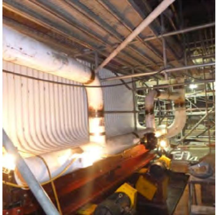
*Lower furnace water walls, downcomers and headers being installed for grate replacement.*
