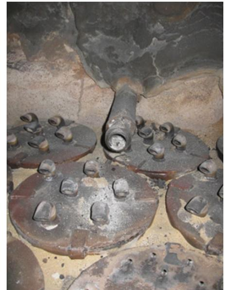
Lower Primary Air Port and Grid Nozzles in Fluidized Bed Boiler
