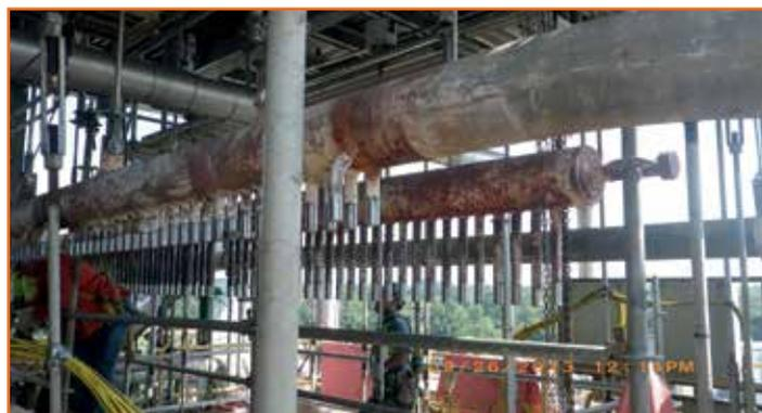
Relocating the primary outlet and secondary inlet headers
