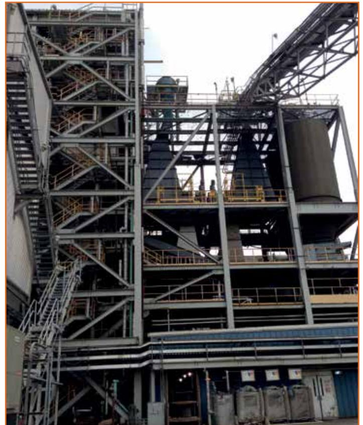
CFB boiler fuel handling system with biomass and waste fuel storage/reclaim bin, coal silos and feeders, drag conveyors, and rotary airlocks
