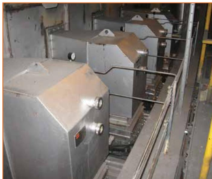
Figure 2: The new OFA nozzle arrangement on the boiler sidewall
