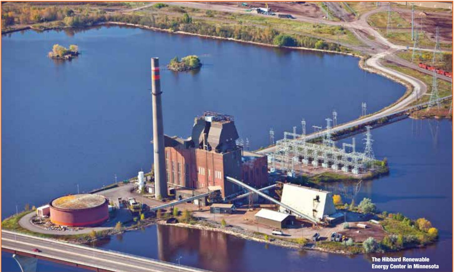
A US-based biomass boiler combustion system specialist reveals how it successfully converted a fossil fuel power station to burn biomass
