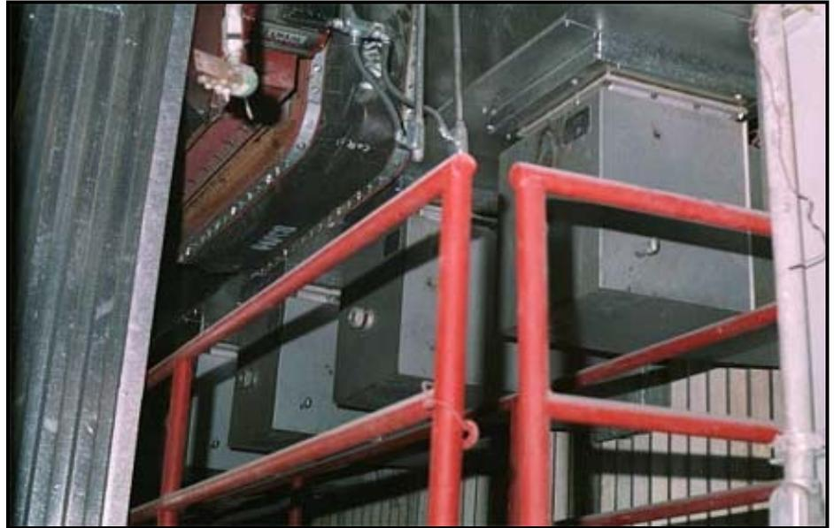
The old “cyclonic” upper air system was removed and ten Jansen High Energy Combustion Air Nozzles™ were installed on the side walls of the furnace (five on the left wall and five on the right wall). The large, aerodynamically efficient nozzles provide high momentum, high energy jets that penetrate well past the center of the furnace.
