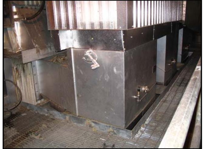
The old overfire air (OFA) system consisted of multiple rows of small OFA ports located on the front and rear walls. A fundamental design limitation that caused insufficient OFA flow capacity and less than optimal mixing of the OFA with the in-flight fuel particles was identified during an in-depth evaluation of the boiler's operation.
