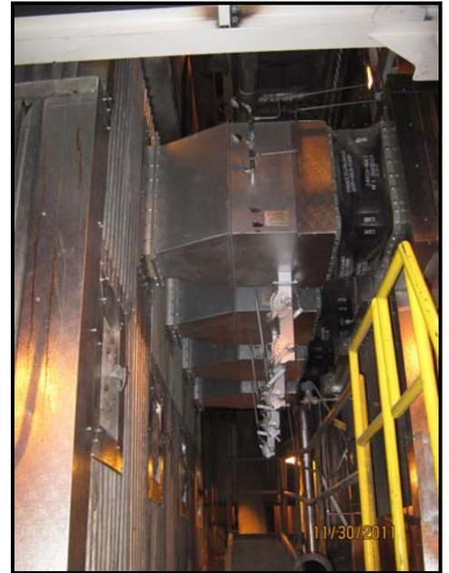
Following an engineering evaluation (including circulation study for generating up to 350,000 lb/hr of steam) and CFD modeling of the boiler, a new JANSEN overfire air (OFA) system was designed and installed in October 2011. At the same time, new fuel distributors were installed to improve the uniformity of fuel distribution over the grate.
