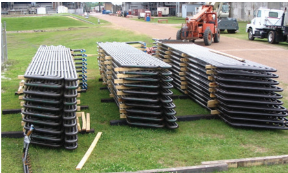
Jansen Superheater Modules Awaiting Installation
