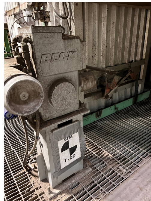
Control Dampers Should Be Set to Automatic Mode
